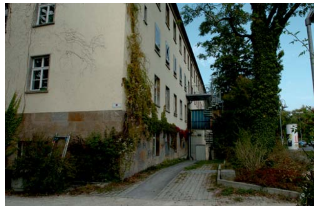
View from rear with backdoor (loading takes place here)
